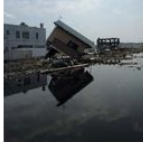
Damage in Kesenuma after tsunami
